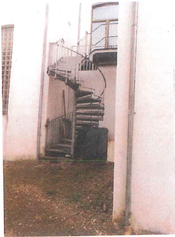
Photo 10; Spiral stairway at rear of 8c West Street
